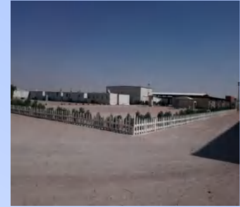
Warehouse in Southern Iraq
